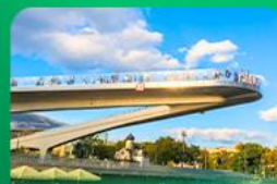
Floating Bridge Moscow
